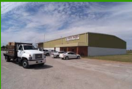
Earth Energy warehouse, Marietta, OK
